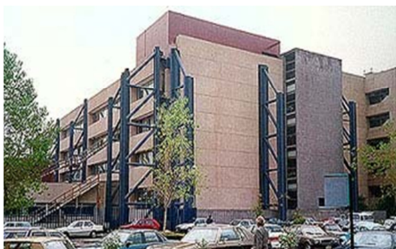
Reinforced Hospital Building (PAHO/WHO)
