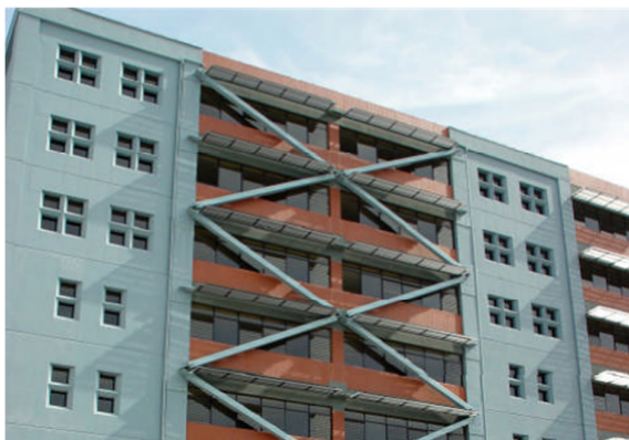
Structurally reinforced hospital, Ecuador (PAHO)
